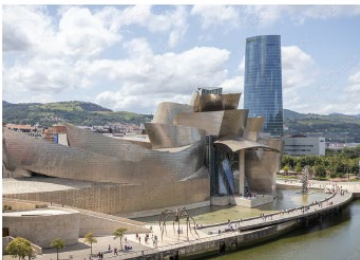
Museum Guggenheim, Bilbao. A cultural building that changed the city's character, 1997, by Frank Gehry.
