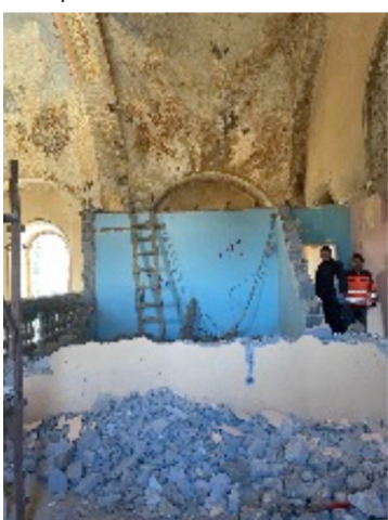
Demolition of inadequate structures
