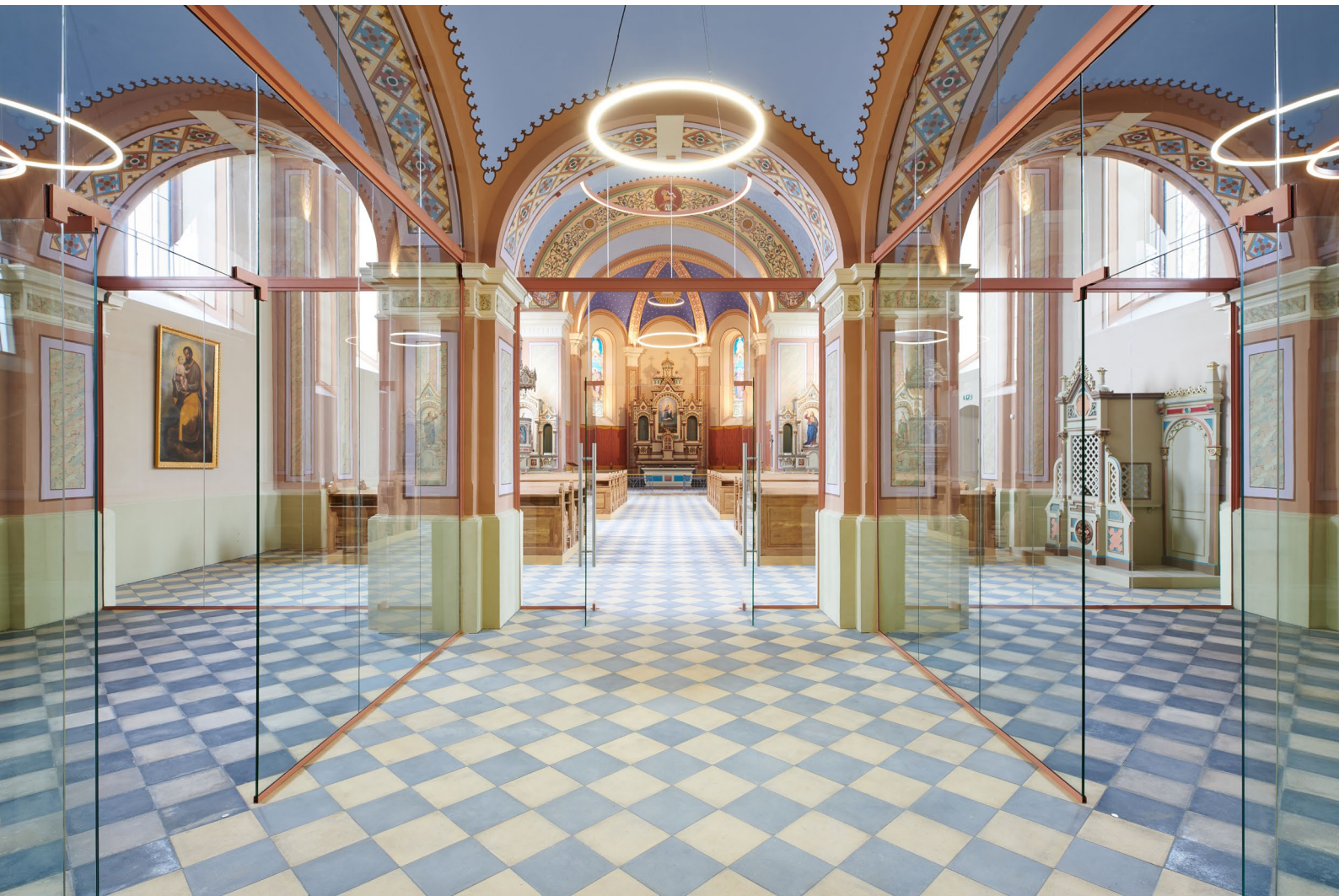
After: Entrance view showing the seamless integration of preserved original floor tiles with newly fabricated elements based on the original pattern.
