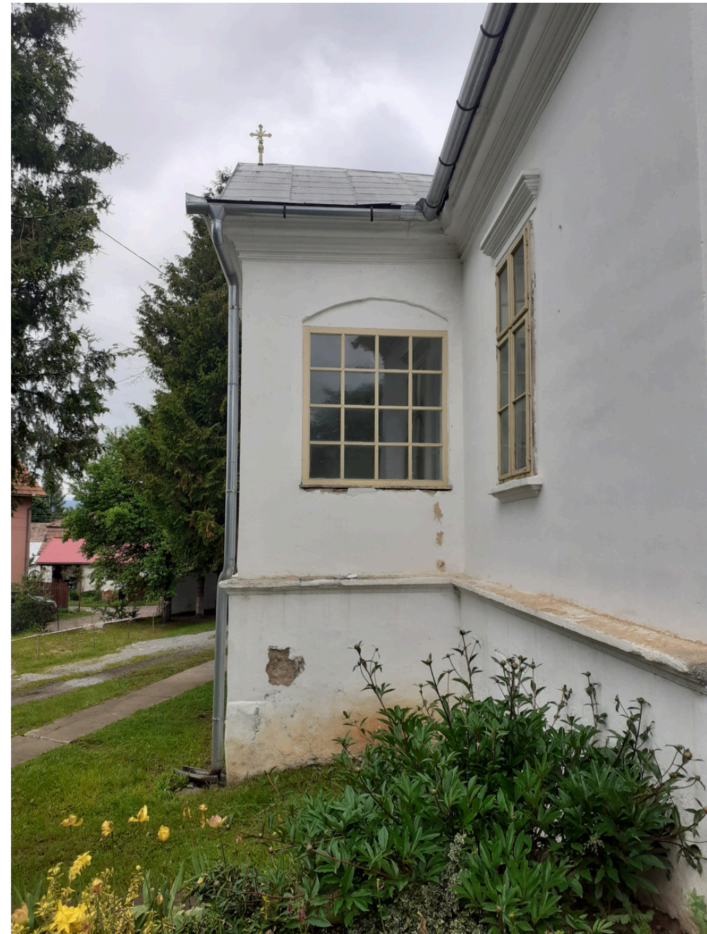
The loggia was closed with a row of windows.
