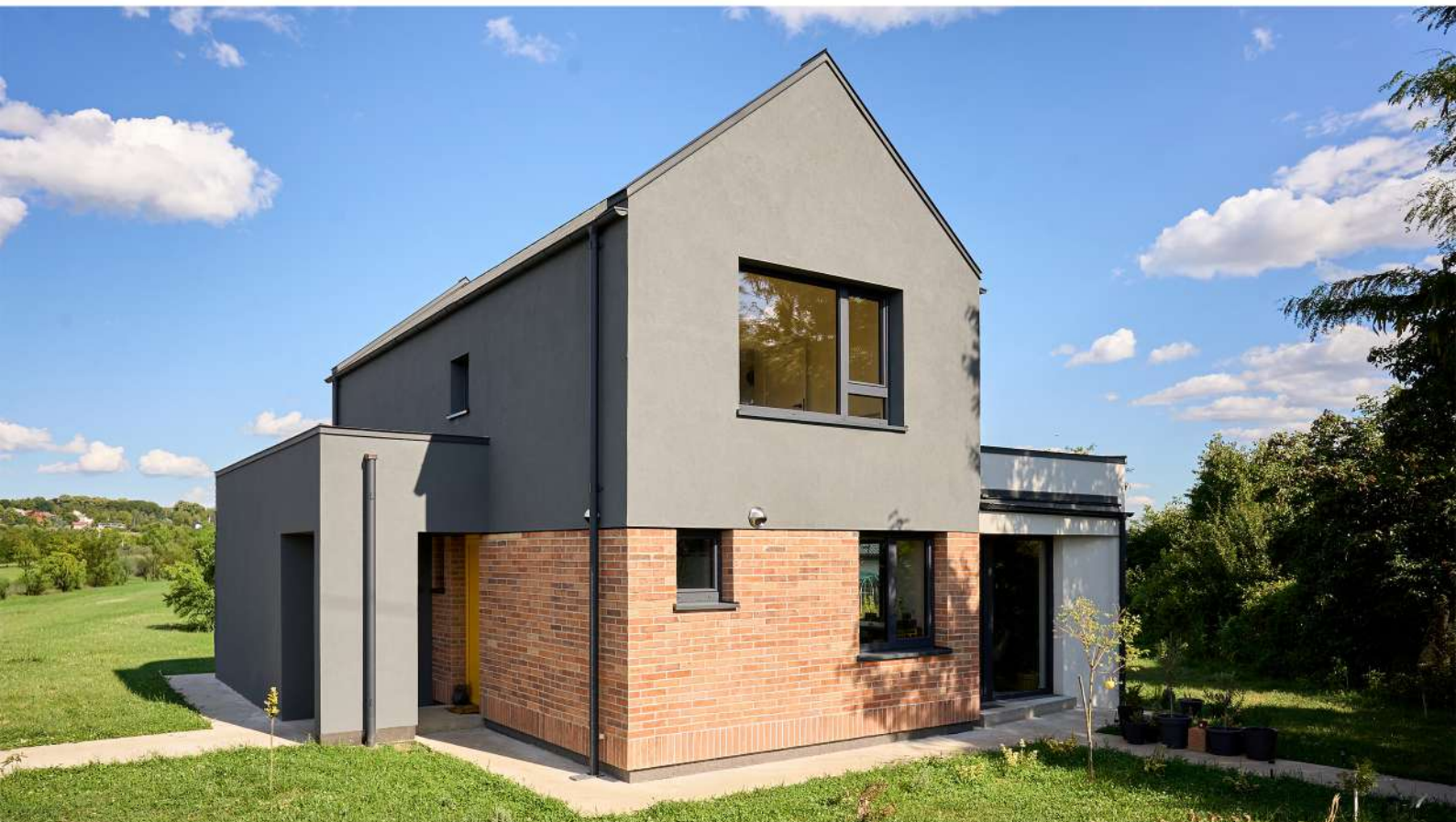
View of the North and West Facades
