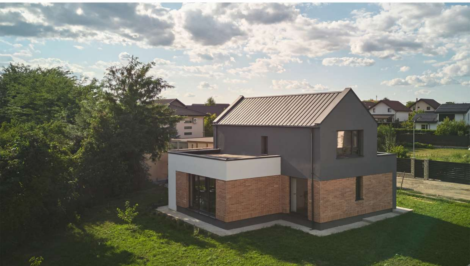
View of the South and East Facades
