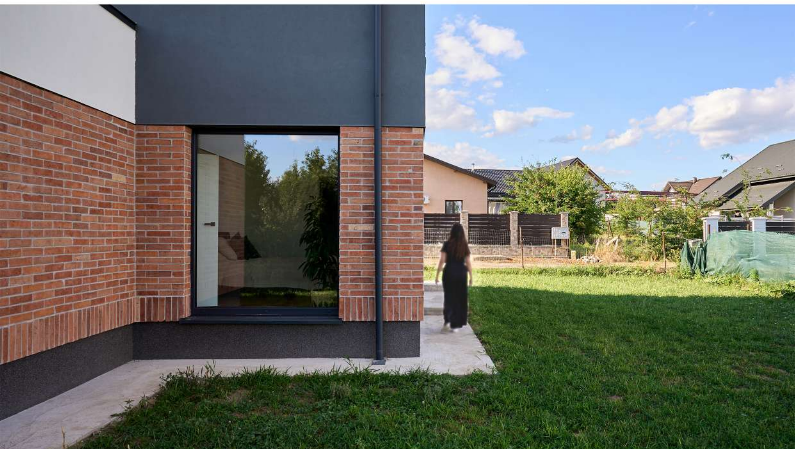
Brick Facade Detail
