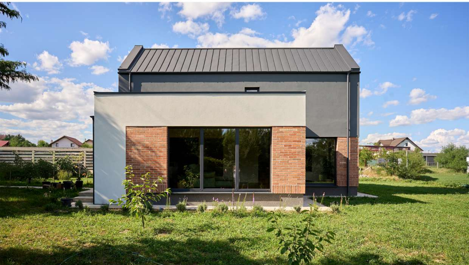
View of the South Facade
