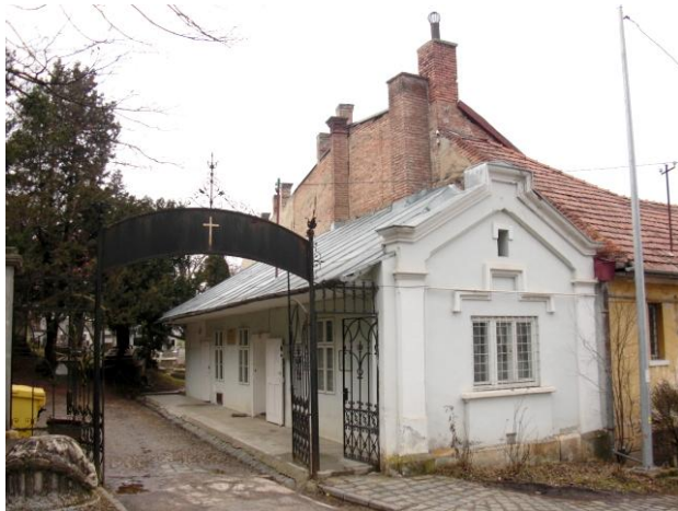
SITE BEFORE INTERVENTION
