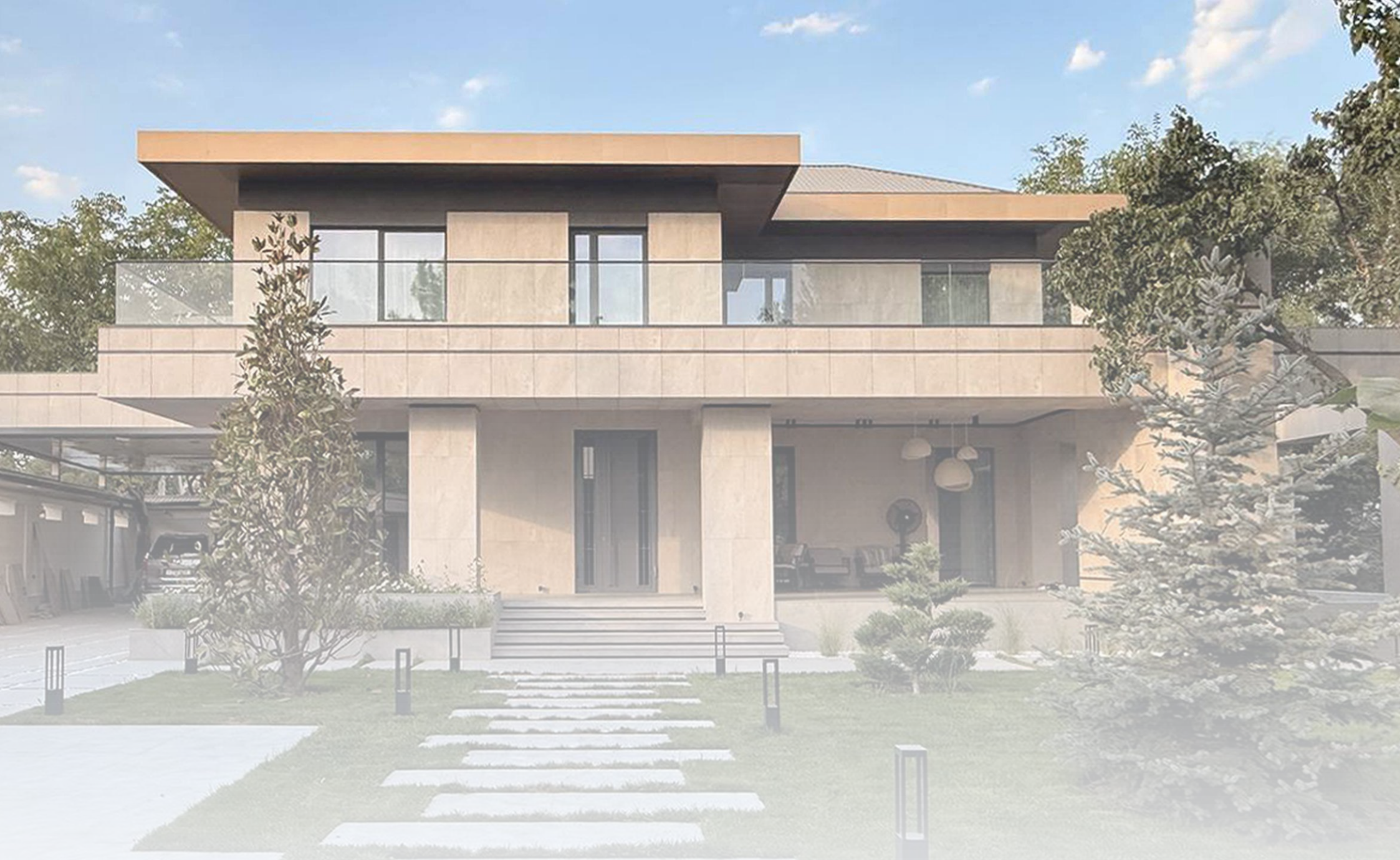
CONTEMPORARY PRIVATE RESIDENCE
