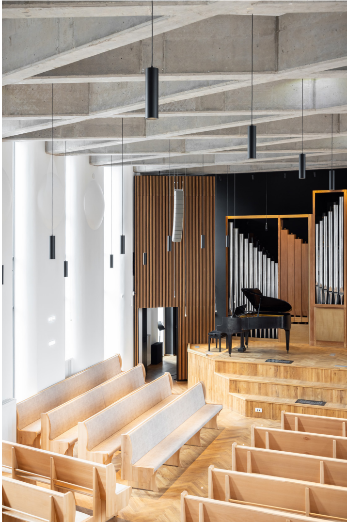
Main hall - exposed concrete coffered ceiling
