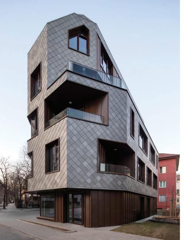
The use of two distinct tones in the material enhances the building's dynamic appearance, with the upper section presenting a more fragmented pattern that casts subtle variations of gray. Highly malleable and durable, titanium-zinc was chosen for both its aesthetic qualities and longevity.
