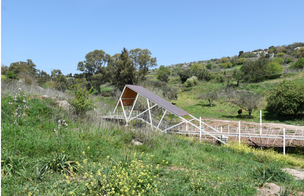
A footbridge over the ravine, bypassing the main trail, acting as a "gateway" to the opposite hillside. Fully reversible structure (steel, wood, copper).
